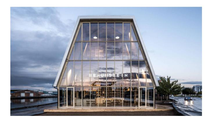
The building uses as few materials as possible, among them Junckers Textured Oak two-strip hardwood flooring. The structure is based on simple tectonic principles, completed with mechanical joints only. As far as possible, building materials used in the construction are not mixed, allowing for removal without contamination and reducing the volume of waste considerably in comparison to similar constructions.
